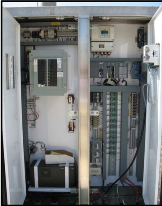
San Sevaine Turnout control panel
