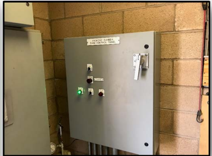
Rubber Dam control panel
